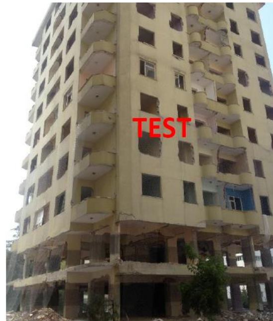
Test Building- Controllably Damaged in one Direction
