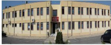
Disaster Coordination Centers / Fire Departments
